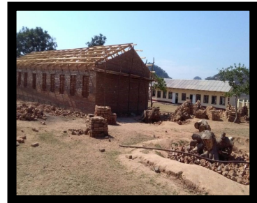
Classroom block under construction
